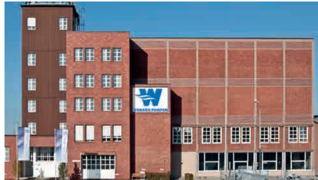
Headquarters building in Wangen, Germany
